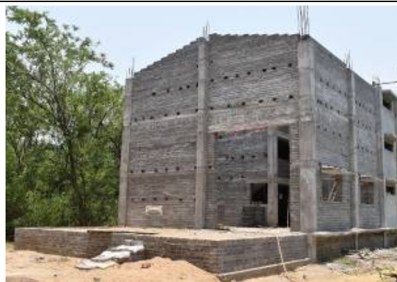
SEED HUB - Infrastructure Development Building work under progress
